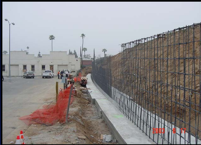
Wall foundation installed – rebar cage under construction
