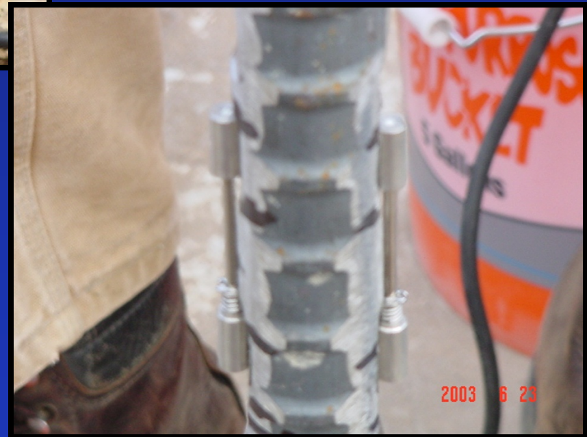
Installed strain gauges (typical)
