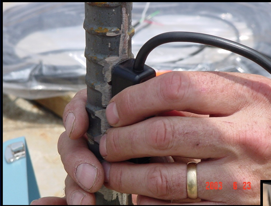
Installation of strain gauge cover
