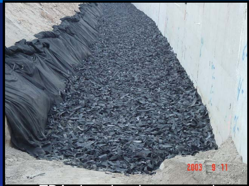
TDA placed and compacted
