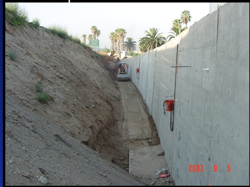
Compaction of foundation soil
