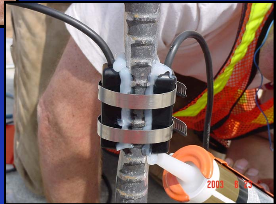
Covers installed and sealed
