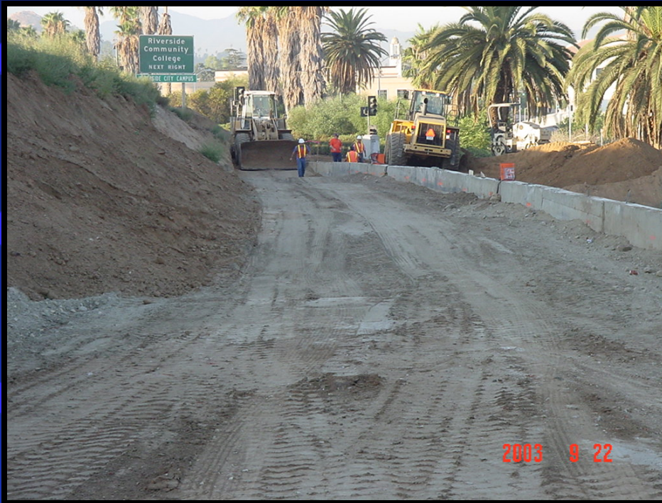
Completed cover soil installation, 2 feet
