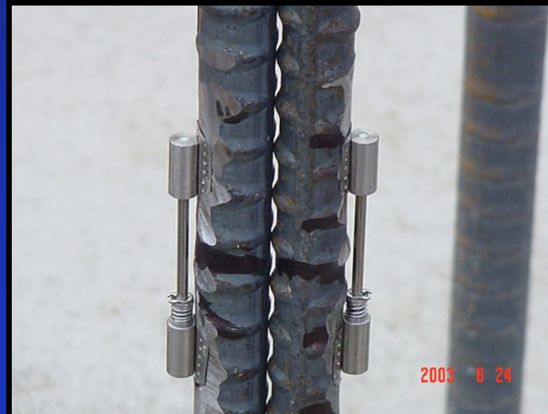
Double rebar install (typical)
