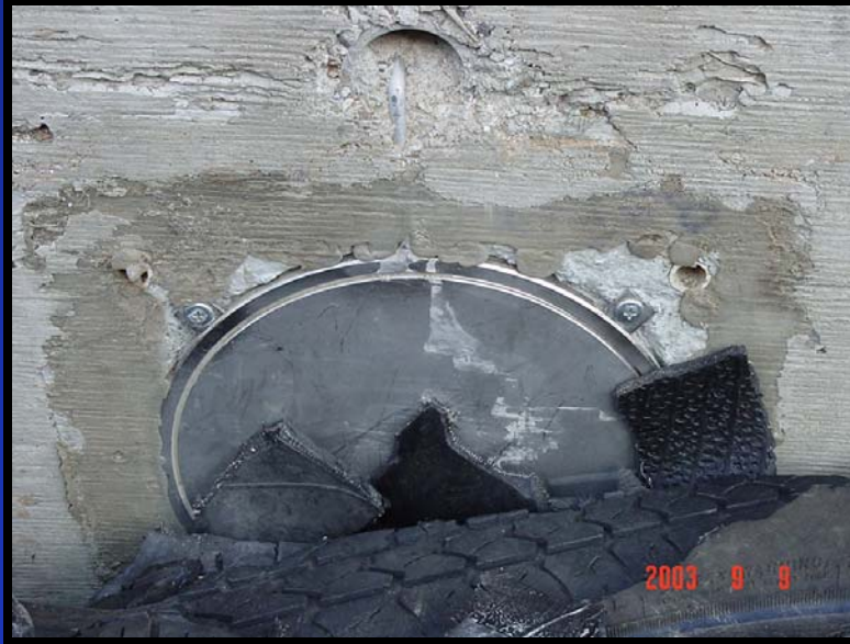
Pressure cell installed
