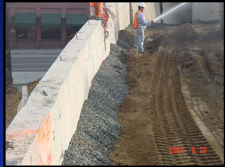
Typical gravel/soil section
