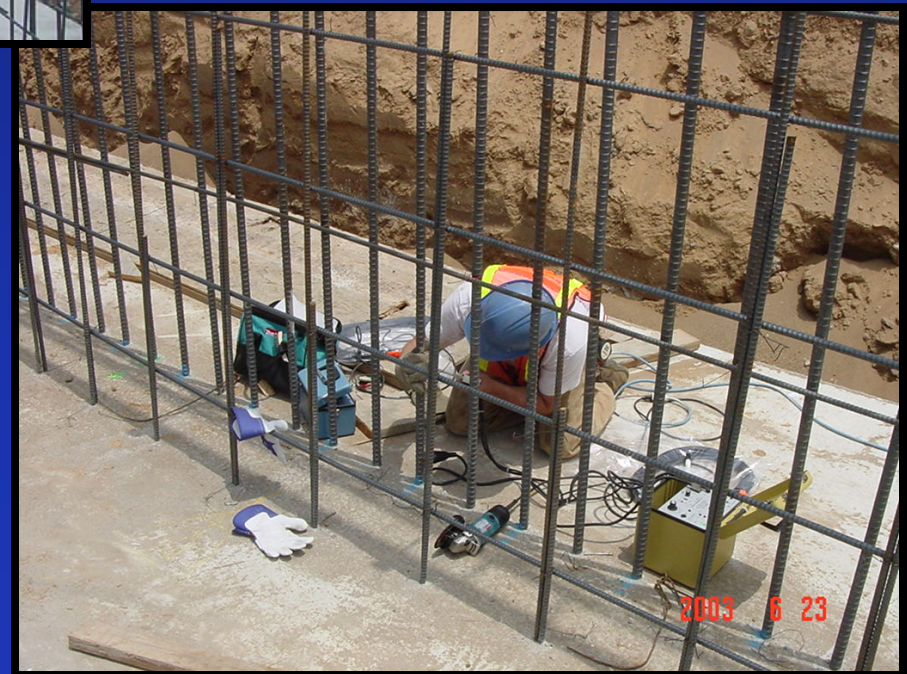
Strain Gauge Installation
