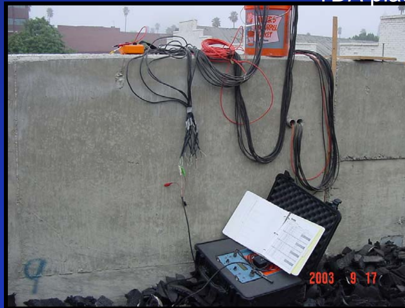
Data collection during construction
