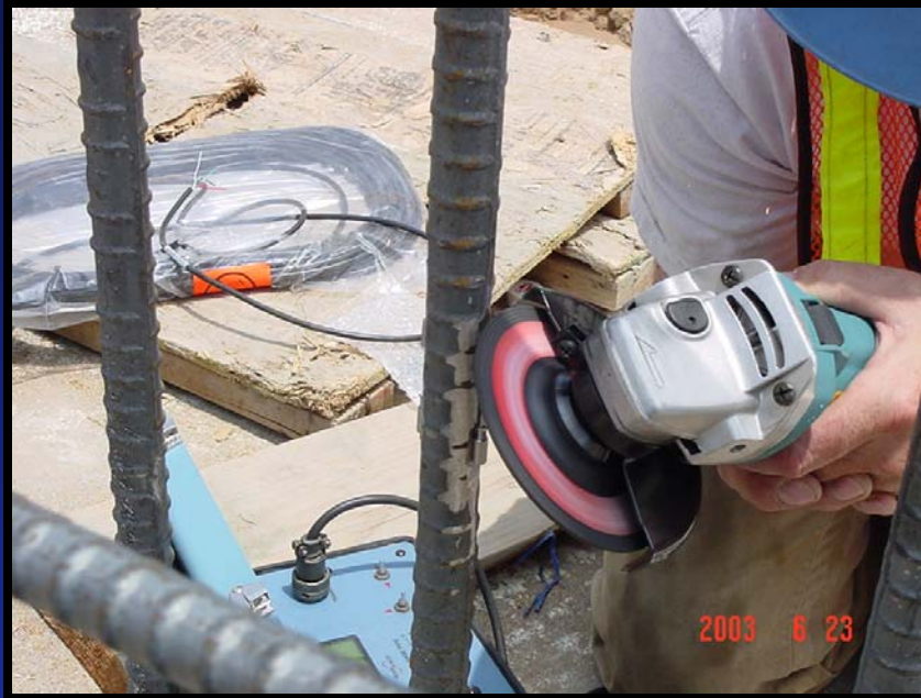
Grinding rebar – Preparation for strain Gauge Installation
