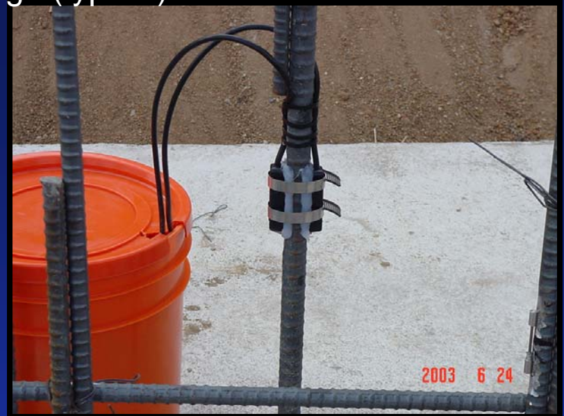
Installed strain gauge (typical)
