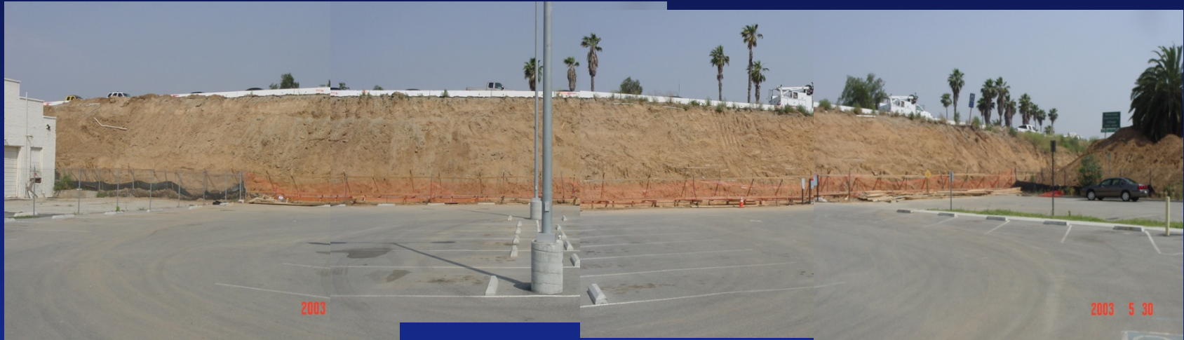
Back-cut of slope prior to retaining wall foundation installation
