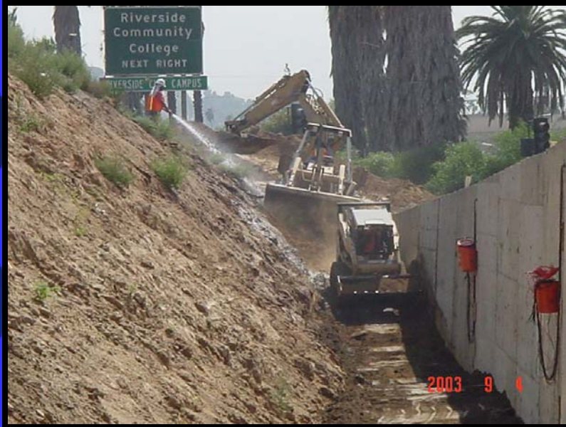
Placement of foundation soil
