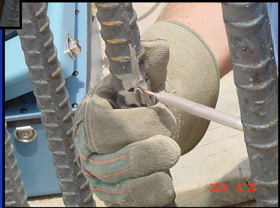
Spot welding strain gauge to rebar
